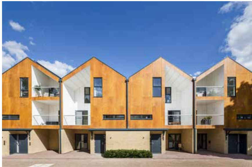
Woodview Mews – Croydon, UK – Geraghty Taylor Architects
